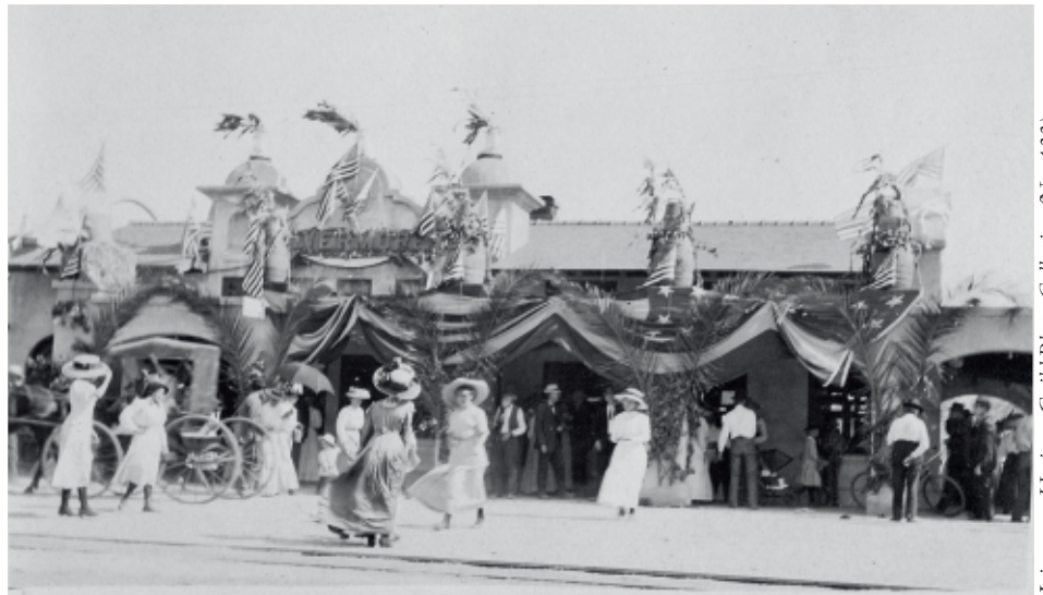
Livermore Western Pacific Railway Co. Passenger Depot was decorated for opening day, August 22, 1910. View is from north, across tracks.
